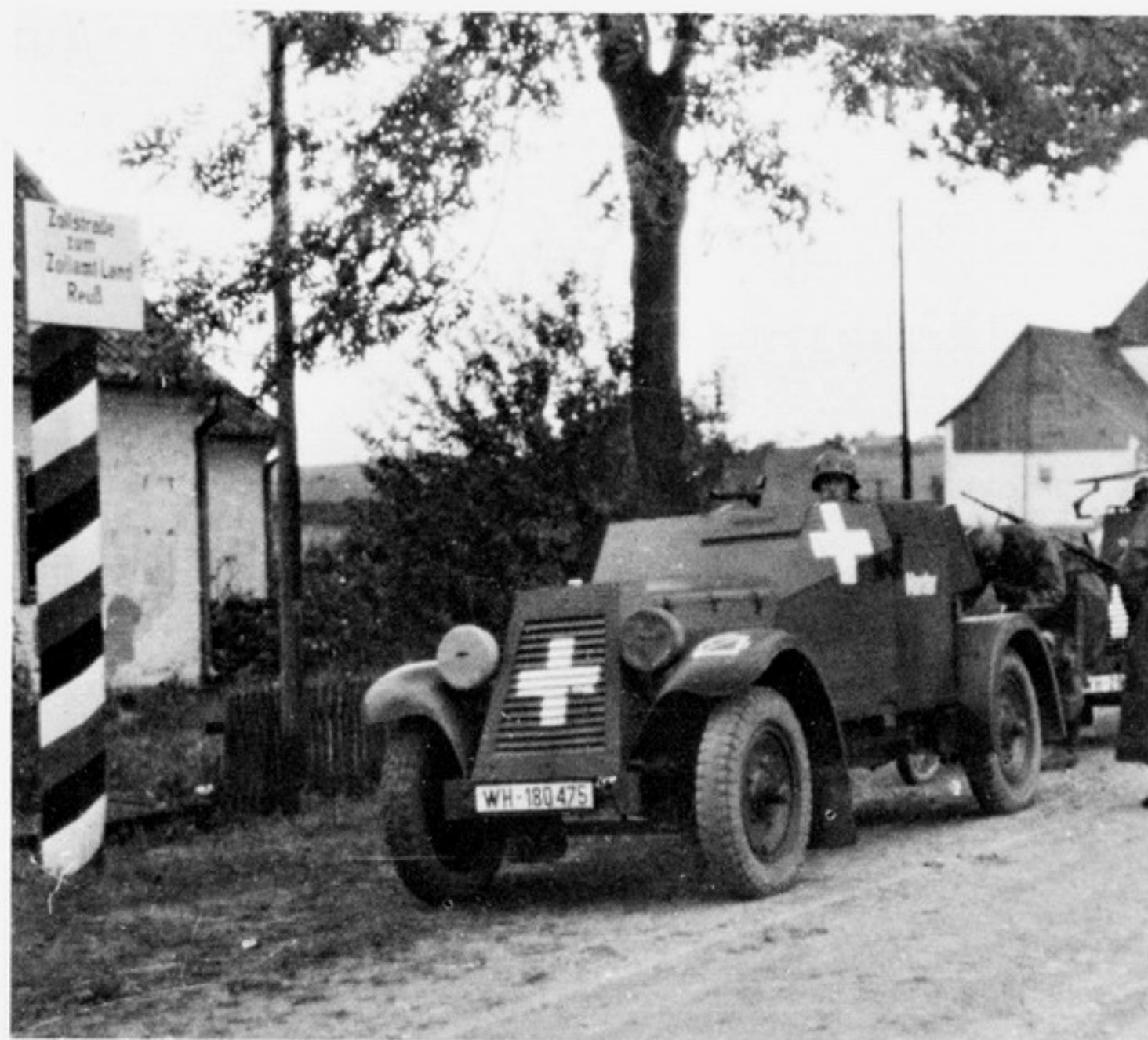
This Adler Kfz 13 MG carrier of a reconnaissance battalion in Poland shows the early white crosses used to identify German combat vehicles. These markings have been painted on, even over the front cooling louvers. All these vehicles have been given names. (Bundesarchiv)
