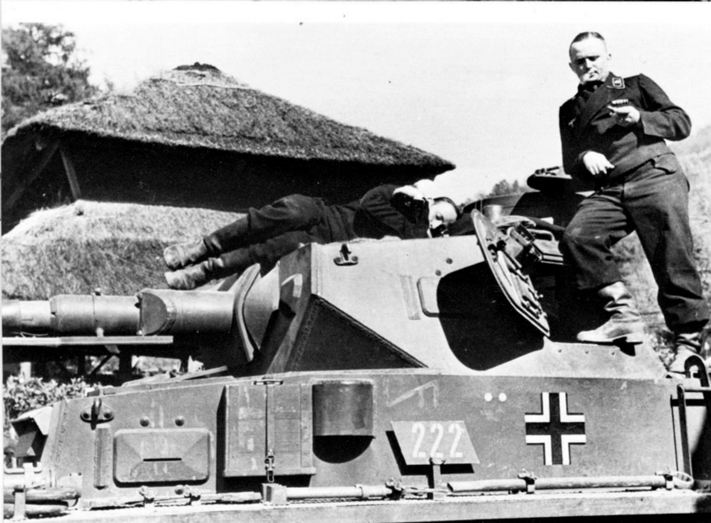
A 2. Panzer Division PzKpfw II ausf C of the signals platoon of II battalion HQ, photographed near Sedan in 1940. The division's 1939-40 sign, 2 small yellow dots, is in front of the cross. The vehicle designator is in white. Note the breaking of the cross out to the antenna trough. (National Archives)
