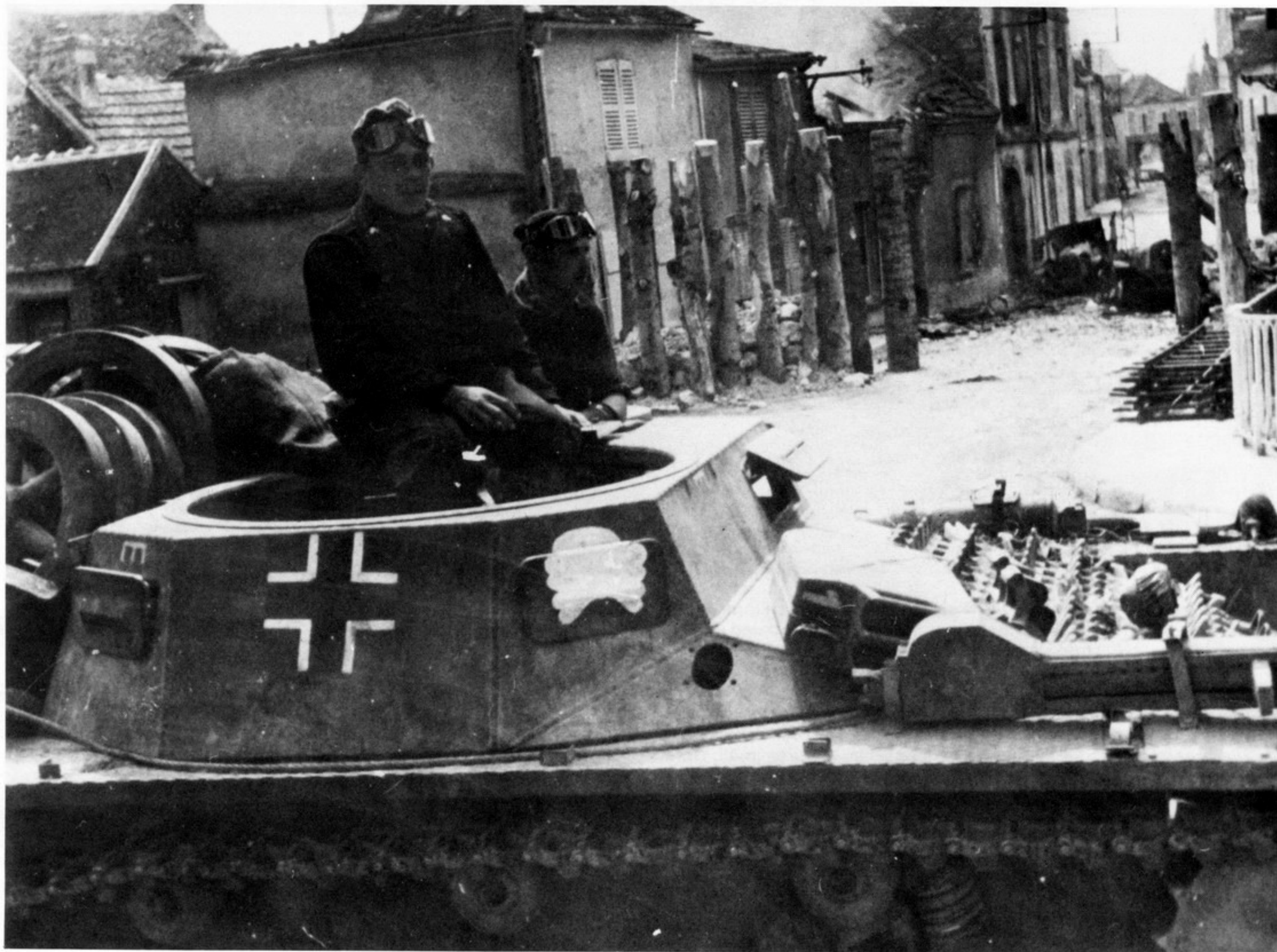
This rare photo shows the 1939-40 sign for 3. Panzer Division. This PzKpfw I ausf. A has been converted into a workshop recovery vehicle. The "Death's Head" ( Totenkopf ) in white was the symbol of all armor troops. The division sign, in yellow, may be a greatly simplified symbol of the Brandenburg Gate in Berlin, the division home station. (National Archives)
